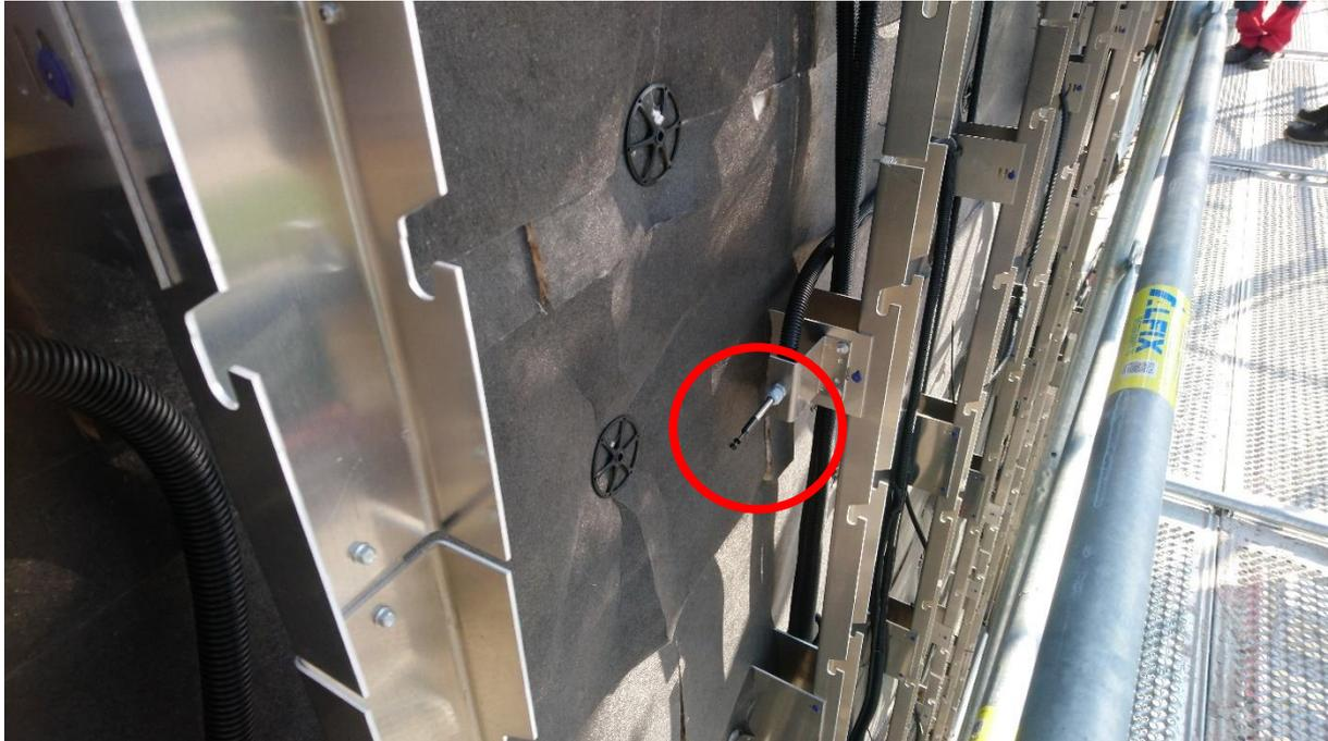
Figure 8: Placement of the air flow measurement device during the construction process
